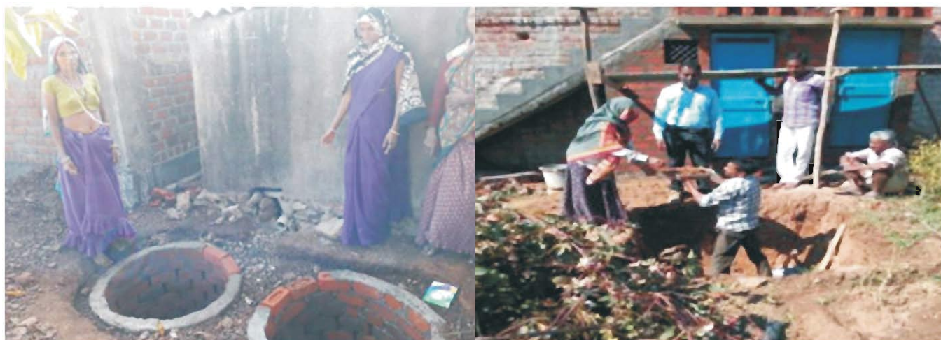
Figure 6: Laying out of dimension for toilet construction and initiating digging of Twin-pit
